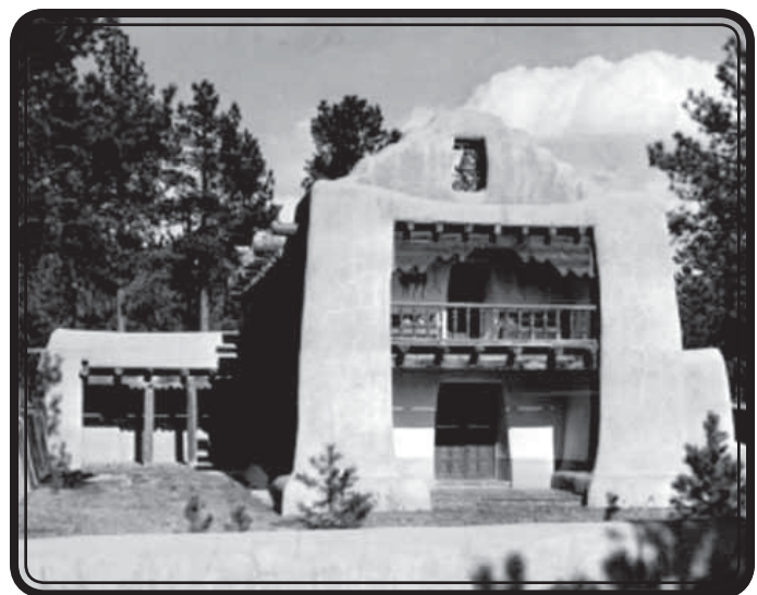
The Taylor Memorial Chapel as it looked in 1929. —Photo: La Foret
